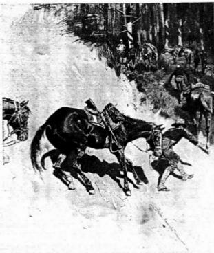
CROSSING A DANGEROUS PLACE.
