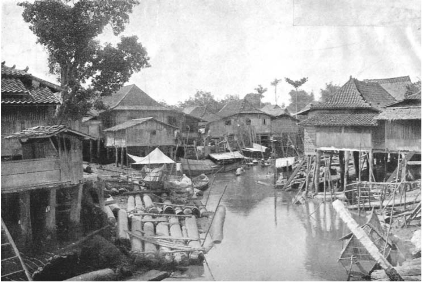
Malayan villages are very much of a piece, with their houses lifted upon piles built along the river bank or water front.
